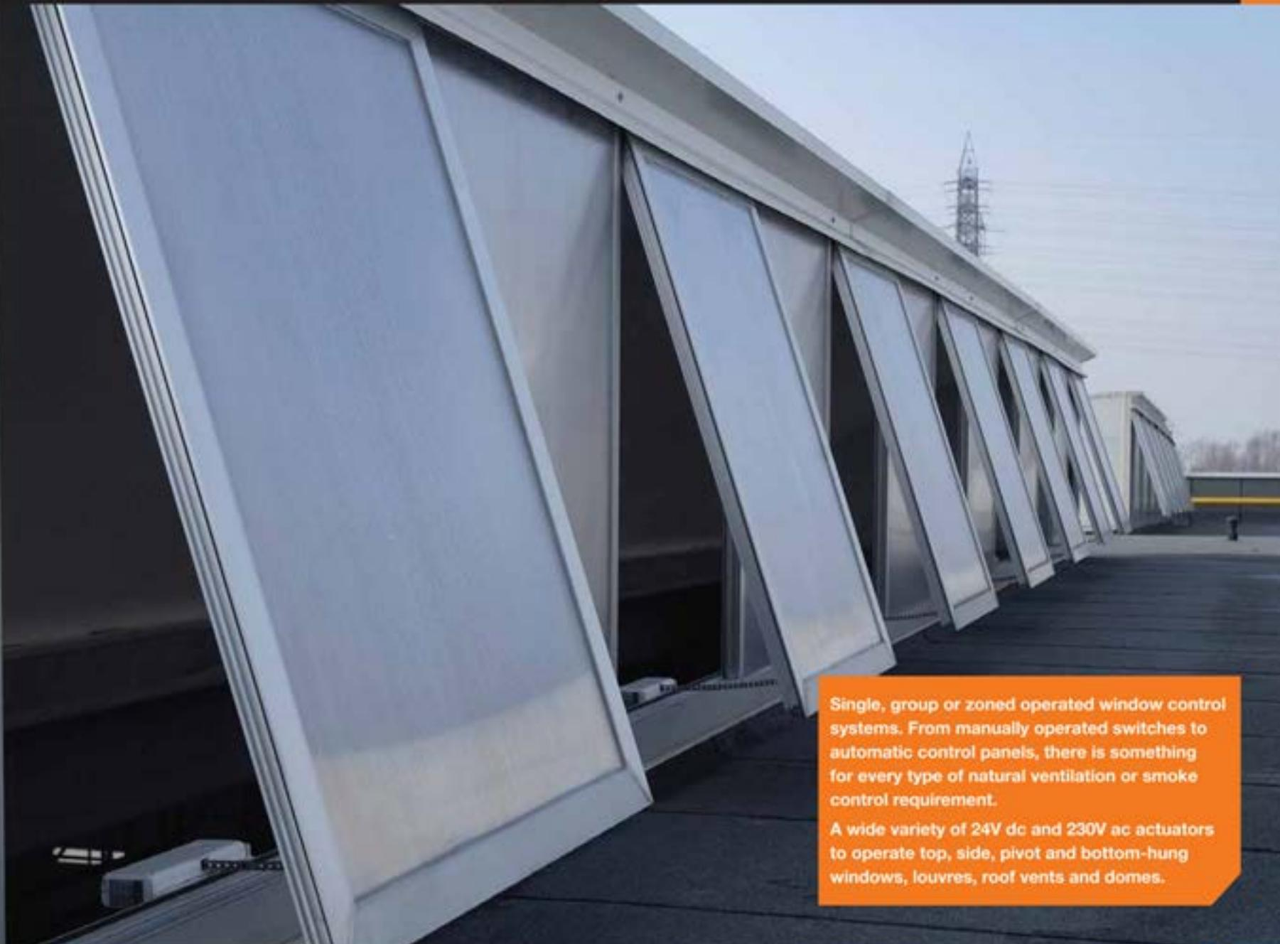
Single, group or zoned operated window control systems. From manually operated switches to automatic control panels, there is something for every type of natural ventilation or smoke control requirement.
