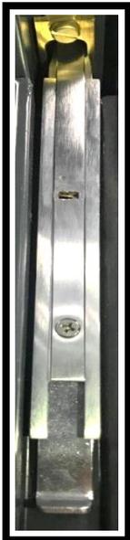
For double leaf doors, there will be a handle and locking system on the master leaf. On the slave leaf, there will be a concealed bolt which will enable the door to remain shut when unused and also have the ability to open and to maximise space. These are key operated. Please see image to the left.
